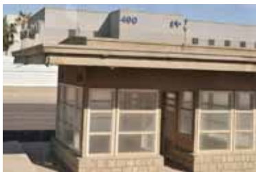
Old Main Gate security office
